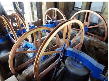
Edward Bishop Chapel on Sunday the 24th. July. The bell frame has been resin-coated, and the final touches for completion should be finished within the next two weeks. These involve installing the clappers, drilling holes for the ropes in the new flooring above the ringing room, and fitting the new ropes, and making the ringing room habitable. The project has been fraught with unexpected problems, necessitating the overall
